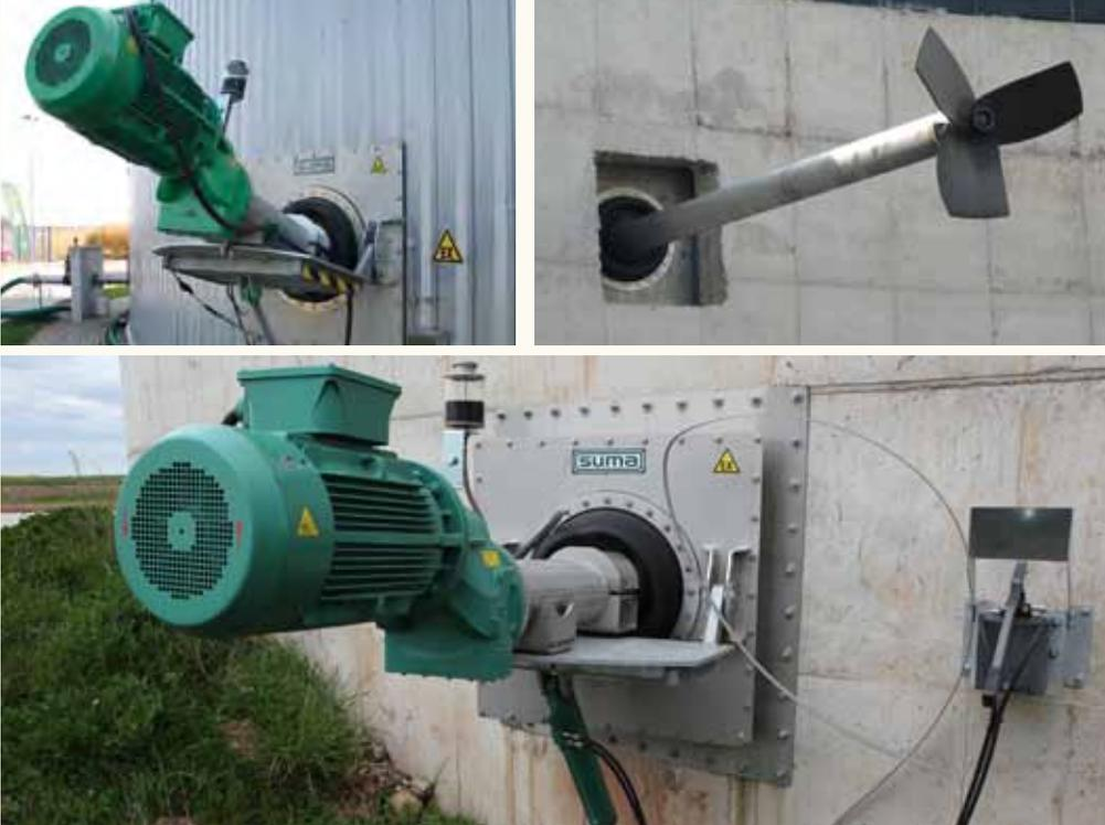
The Giantmix AMT is used for larger fermenter, post digester and gas-tight end storage tanks.
