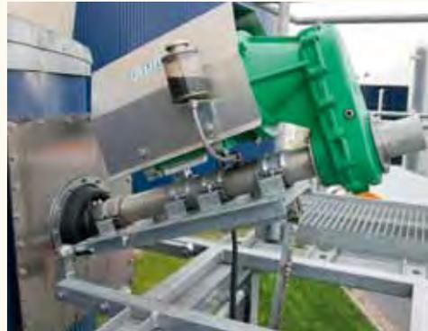
For technical reasons due to loads, the Giantmix FR cannot be directly mounted to the wall of a steel digester.
